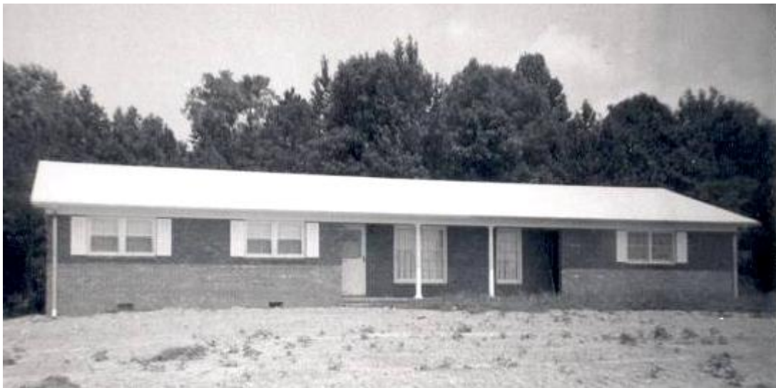
The "New Parsonage" - built 1971
